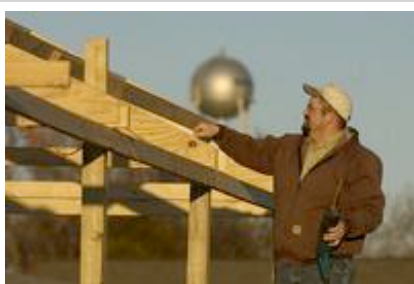
(AP) Dean Krehbiel works on a shed behind his new home which is being built in Marquette, Kan. Thursday,...
